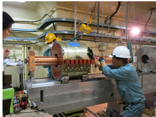
Figure 3: LAS structure insertion into DC solenoid.
