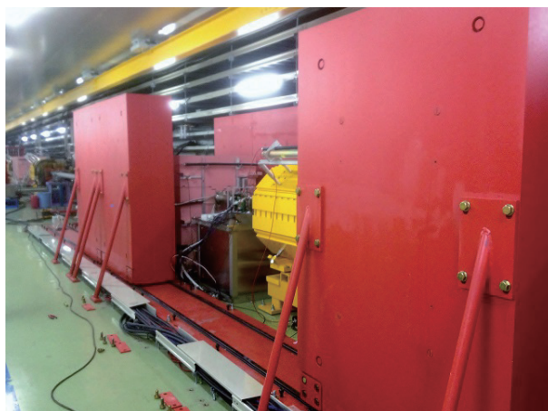
Figure 4: Collimator section. The power FETs and RadMon are located on the desk downstream of the beam collimator. The collimator, the desk and quadrupole magnets near the collimator are covered by the movable shielding.
