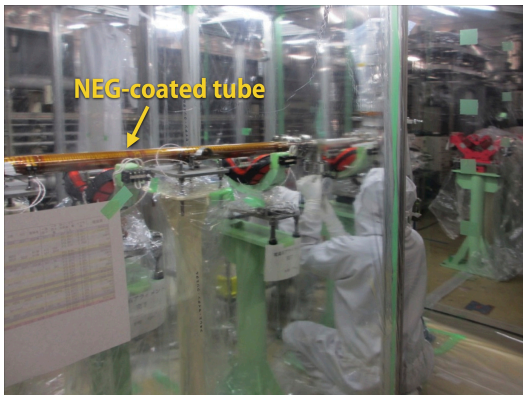
Figure 3: Installation of a NEG-coated beam pipe near the SC main linac.
