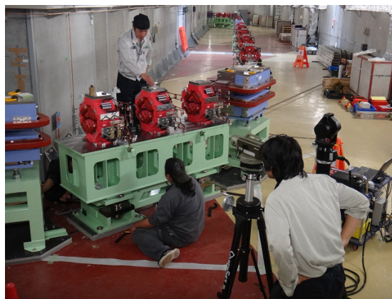
Figure 2: Magnet installation and alignment.
