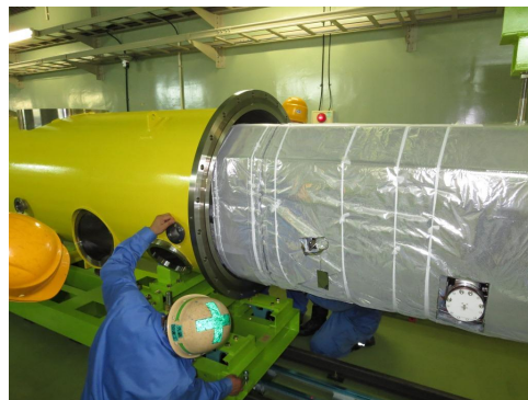
(a) Assembly of vacuum vessel
