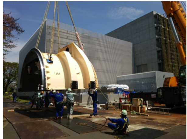
Figure 7: Installation of the gantry structure to the gantry room in NIRS. [6]
