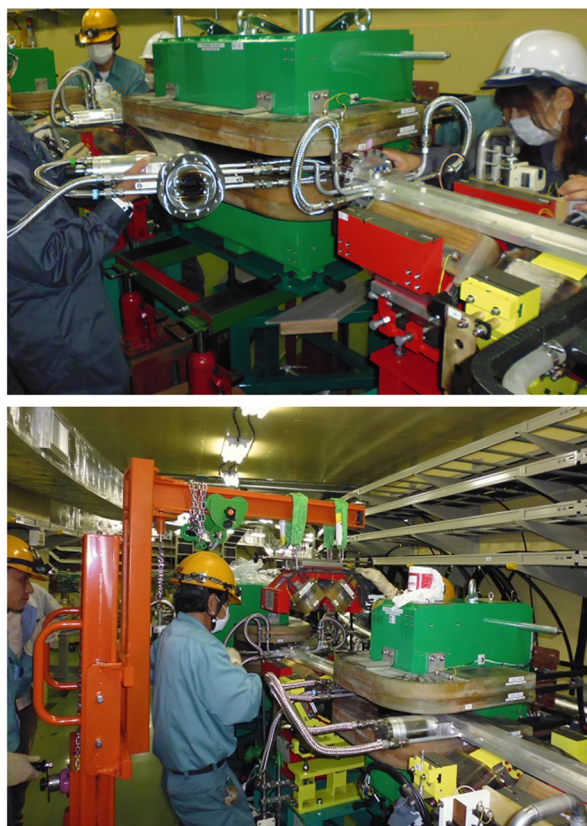
Figure 7: Installation of the beam duct into the arc section.
