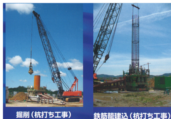
Figure 4: Piles installation.
