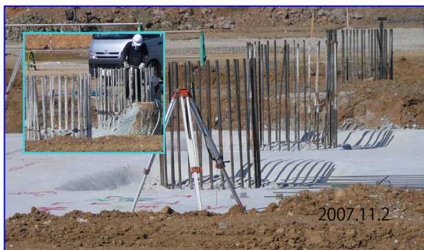
Figure 5: Scraping pile after installation and three lines of piles.
