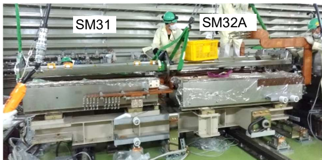
Figure 3: Disassembly of SM31 and SM32A/E.
