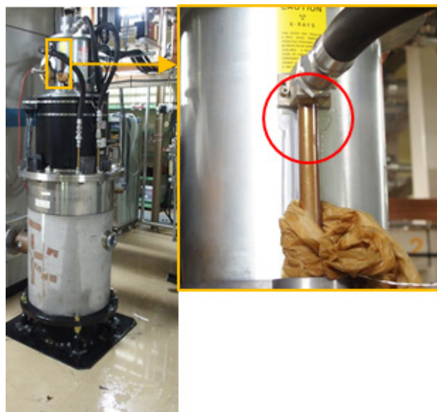
Figure 2: Water leak point.
