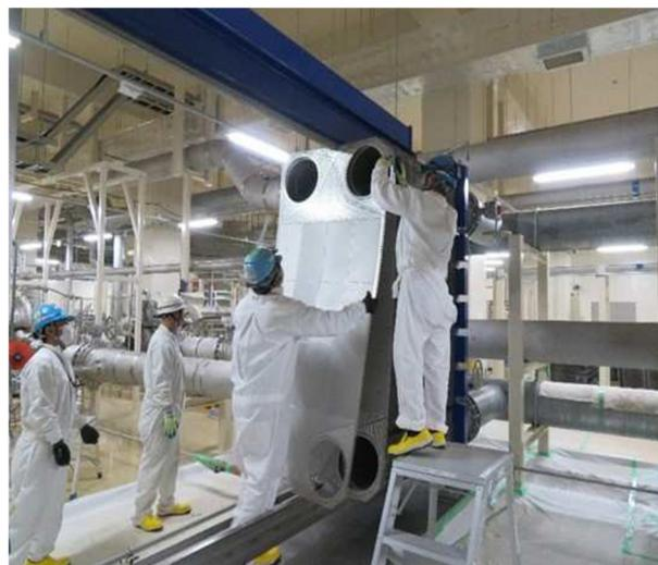
Figure 5: Disassemble of the exchanger plates.
