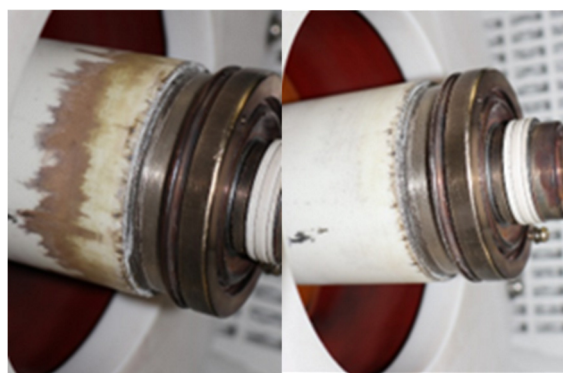
Figure 5: Insulators before and after cleaning.
