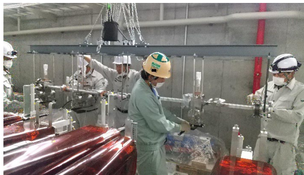
Figure 5: Installation of vacuum chamber.
