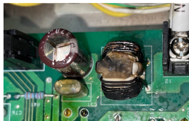
Figure 5: Damage to the auxiliary power supply board.
