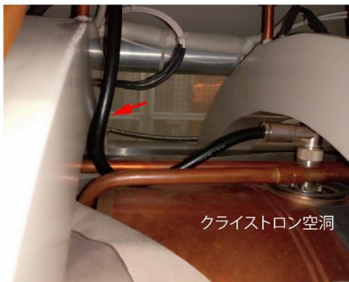
Figure 8: An RF leakage point at the RF inlet of the klystron. A schematic drawing and a photograph are shown in top and bottom, respectively. A leakage was found at a short cable to the klystron cavity as indicated by a red arrow in the bottom.
