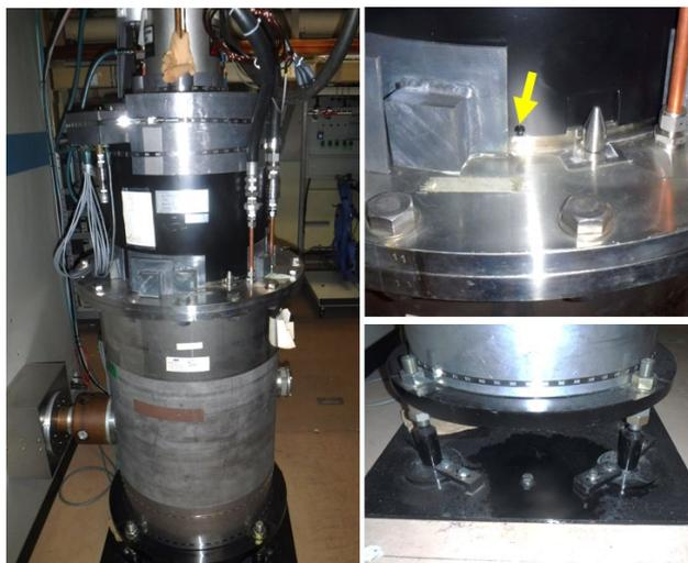
Figure 2: Water leakage from Klystron magnet.
