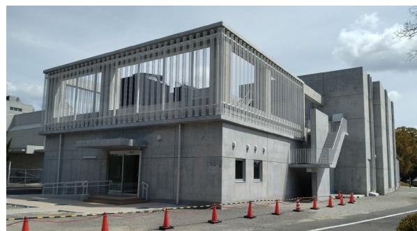
Figure 2: Photo of the TAT cyclotron building.
